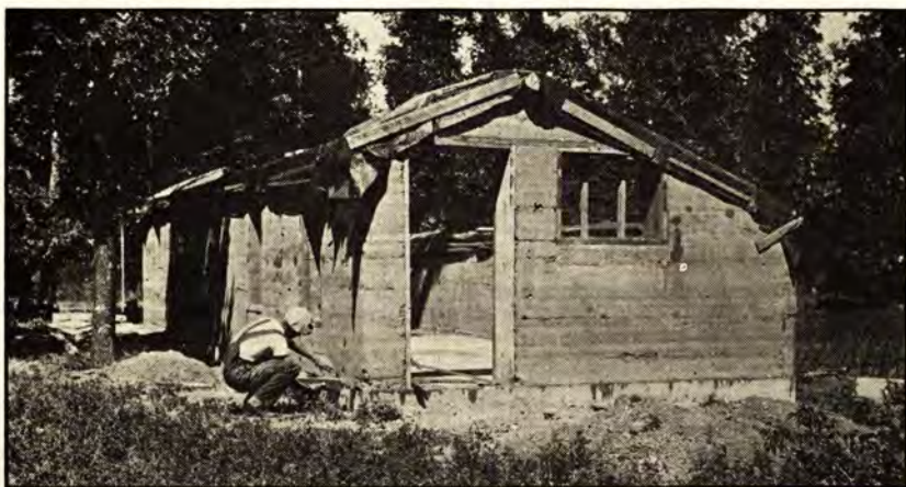
Figure 34.—PROTECTING THE TOP OF RAMMED EARTH WALLS DURING CONSTRUCTION.
