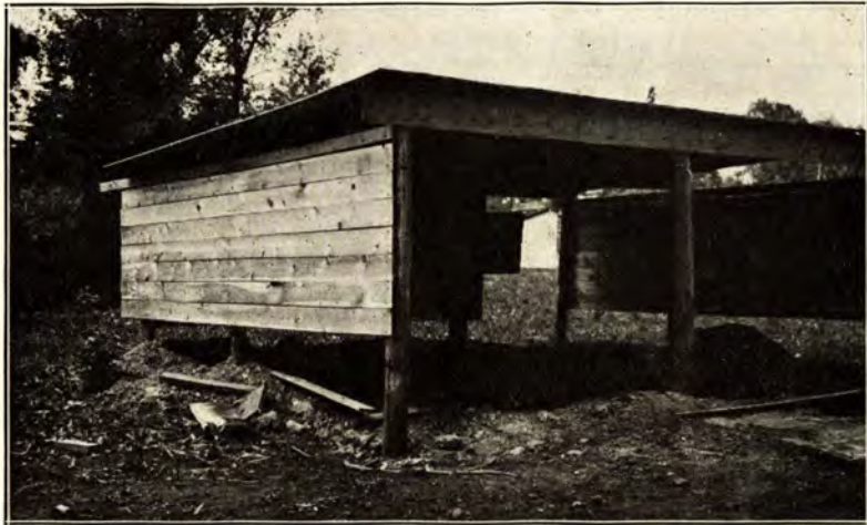
Figure 23.—A SHELTER FOR PROTECTING THE SOIL USED FOR RAMMED EARTH WORK.
