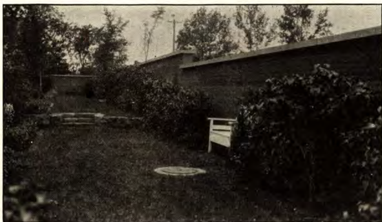
Figure 19. —THIS GARDEN WALL OF RAMMED EARTH WAS BUILT IN 1934 AND WAS STUCCOED IN 1935.
