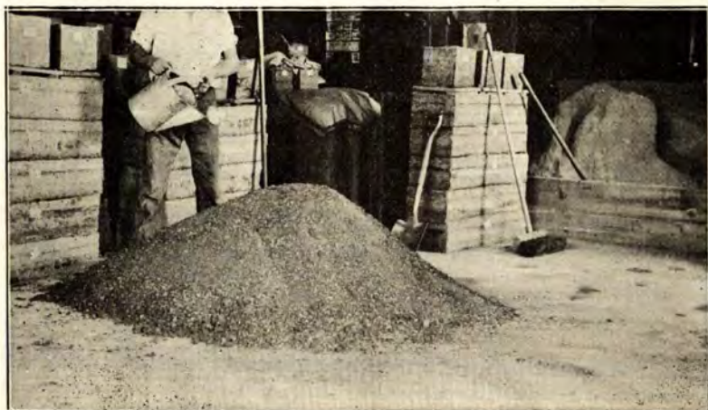
Figure 14.—ADDING MOISTURE TO DIRT FOR RAMMED EARTH WORK.
