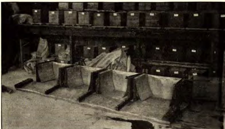
Figure 37. —A FORM FOR MAKING BUILDING BLOCKS OF RAMMED EARTH.
