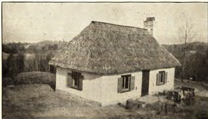
Figure 47.—A DWELLING HOUSE WITH PISE' WALLS AND THATCHED ROOF.
