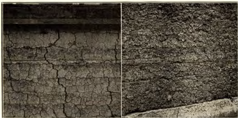
Figure 13.—AN EXPERIMENTAL WALL OF HEAVY CLAY OR "GUMBO" SOIL.
