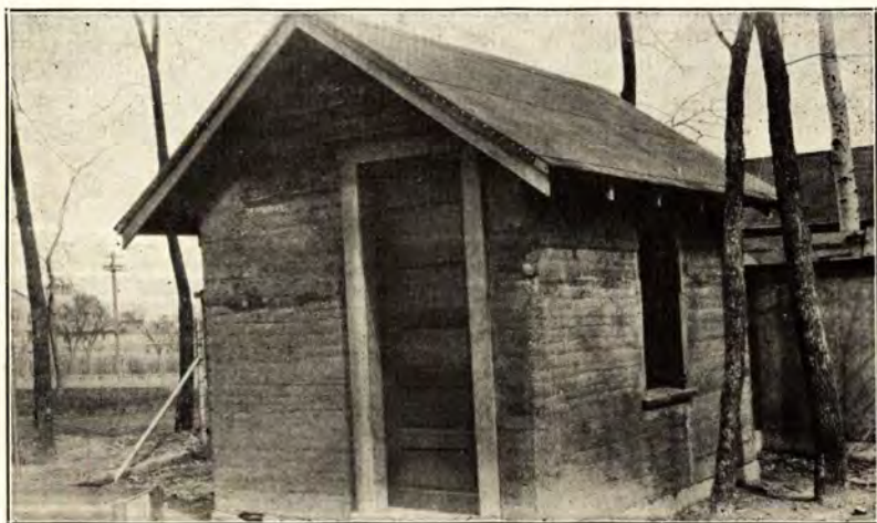
Figure 17.—A SMALL RAMMED EARTH BUILDING USED FOR EXPERIMENTAL PURPOSES.
