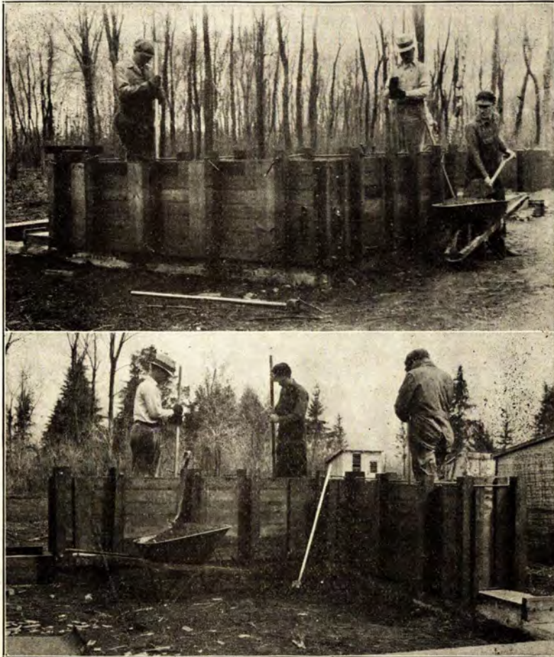
Figure 30.—RAMMED EARTH WALL FORMS LEVELED AND CLAMPED TO THE CONCRETE FOUNDATION
