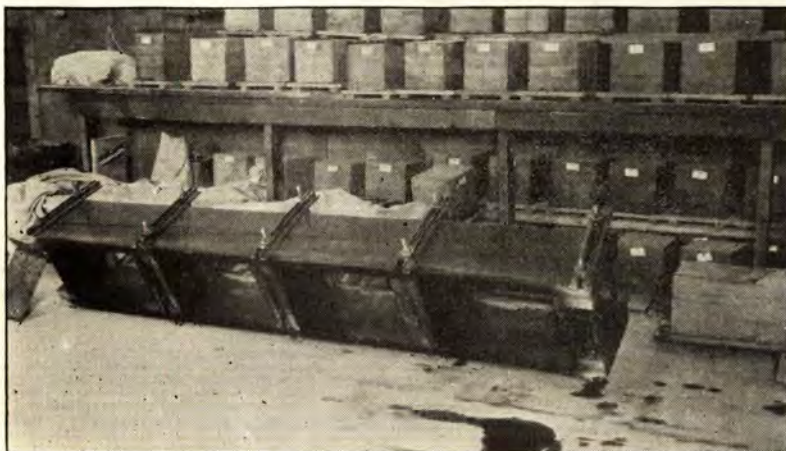
Figure 38. —A FORM WITHOUT A BOTTOM FOR MAKING BUILDING BLOCKS.
